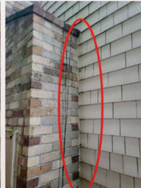
Wood decay next to the masonry chimney
